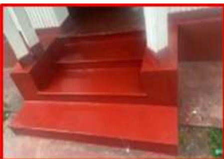
Even the front steps received a coat of paint.
