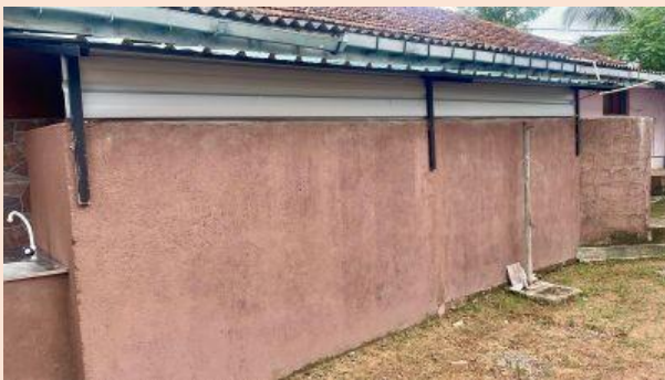
The back wall has had a coat of paint
