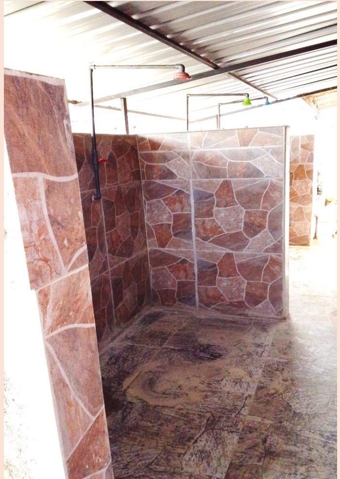
New shower heads fitted
