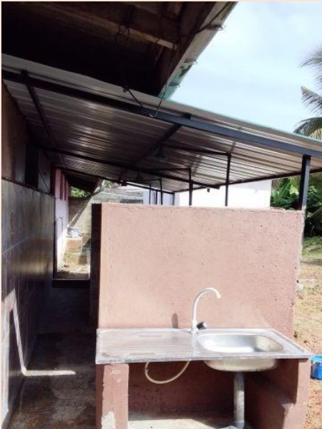
The roof was fitted first
